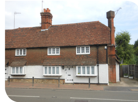
Clay tile roof and tile-hanging
