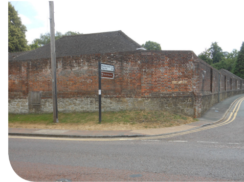
Kentish ragstone and brick walls
