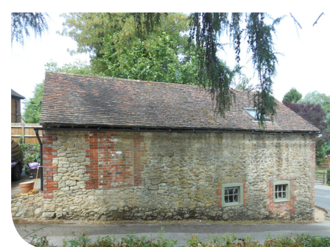
Rubble stone walls
