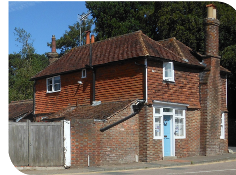
Clay tile roofs and tile-hanging
