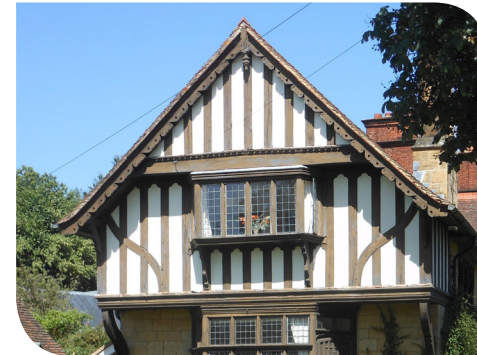
Steeply pitched roofs
