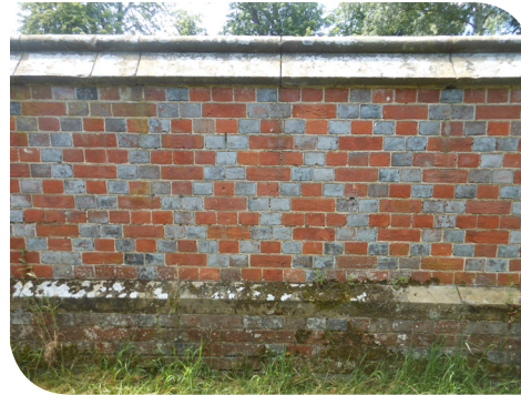
Brick estate wall to Hall Place
