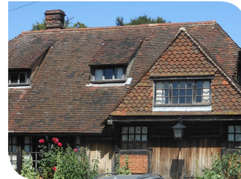
Clay tile roofs and tile-hanging
