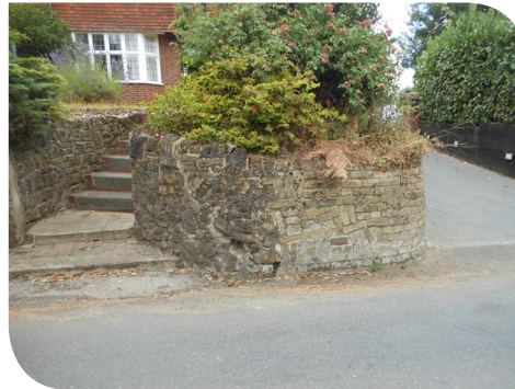
Stone and brick retaining wall
