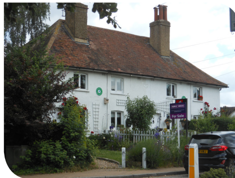
Unbroken roof slopes
