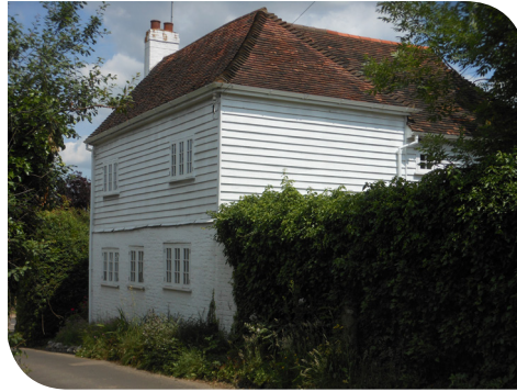
Weatherboarding and brick covering timber frame
