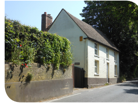
Unbroken roof slopes
