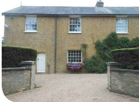
Yellow brick and slate roofs
