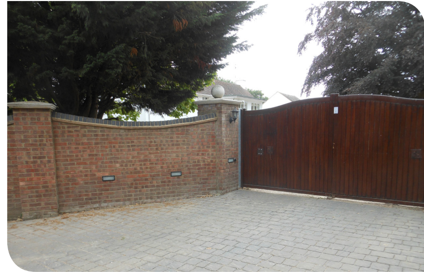
Modern boundary treatment of inappropriate suburban character
