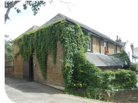
Yellow brick and slate roofs
