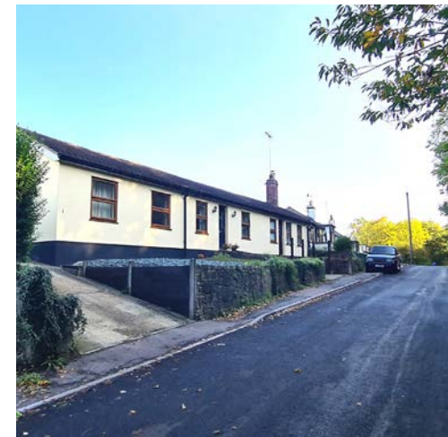
Figure 30: Bungalows with access from the street and a view to the Green Belt from the back gardens.
