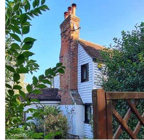
Figure 62: Brick chimney connected to the ground.
