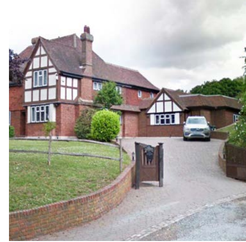
Figure 76: Single-storey side extension.
