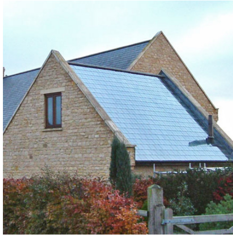
Figure 88: Solar panels integrated sympathetically with a traditional building.
