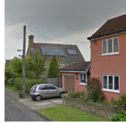
Figure 89: Solar panels integrated with a contemporary design in New Swanley Village.
