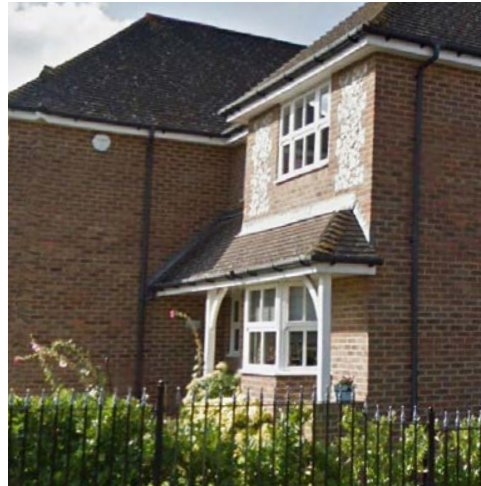
Figure 71: Bay window under a pitched porch.
