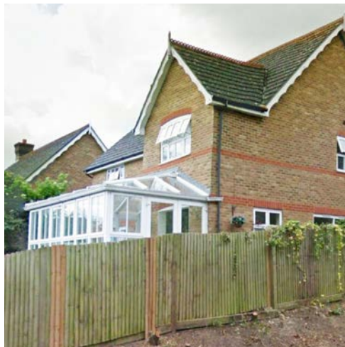
Figure 77: Single-storey rear conservatory extension.
