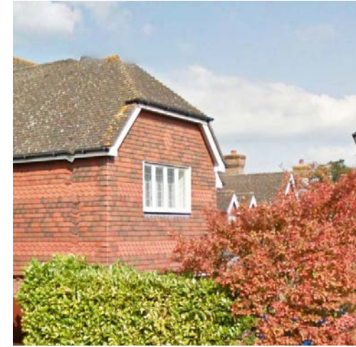
Figure 86: Vertical hung tiles used on facade of the building.
