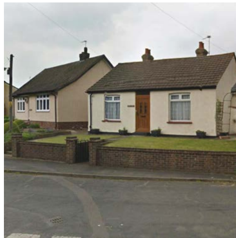
Figure 43: Low retaining wall at the boundary of the front garden.
