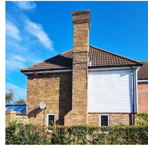
Figure 65: Contemporary building with a brick chimney connected to the ground.
