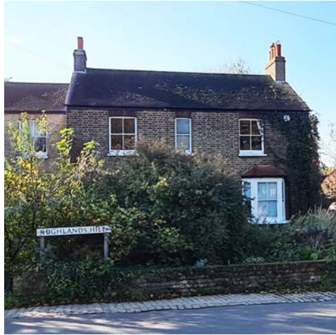
Figure 60: Pitched roof with symmetrical chimneys.
