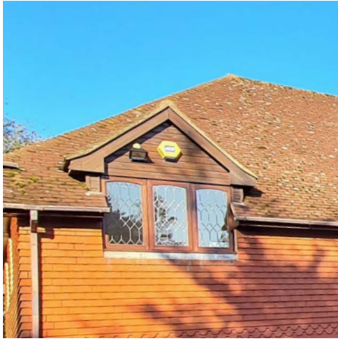
Figure 67: Dormer window within the Conservation Area.
