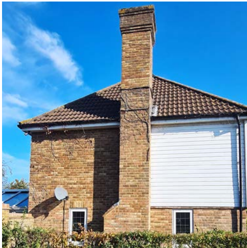
Figure 84: Characteristic white weatherboard and yellow bricks.
