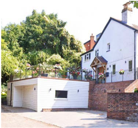
Figure 81: Traditional white weatherboarding used to create a contemporary finish.
