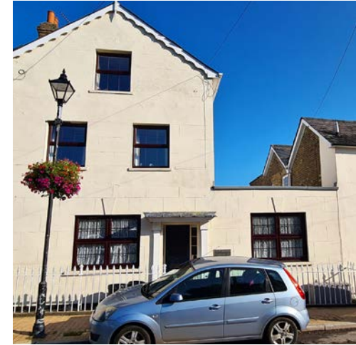
Figure 27: Building fronting onto the road.
