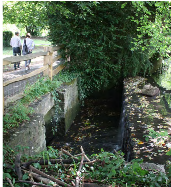
Sluice within the central lake
