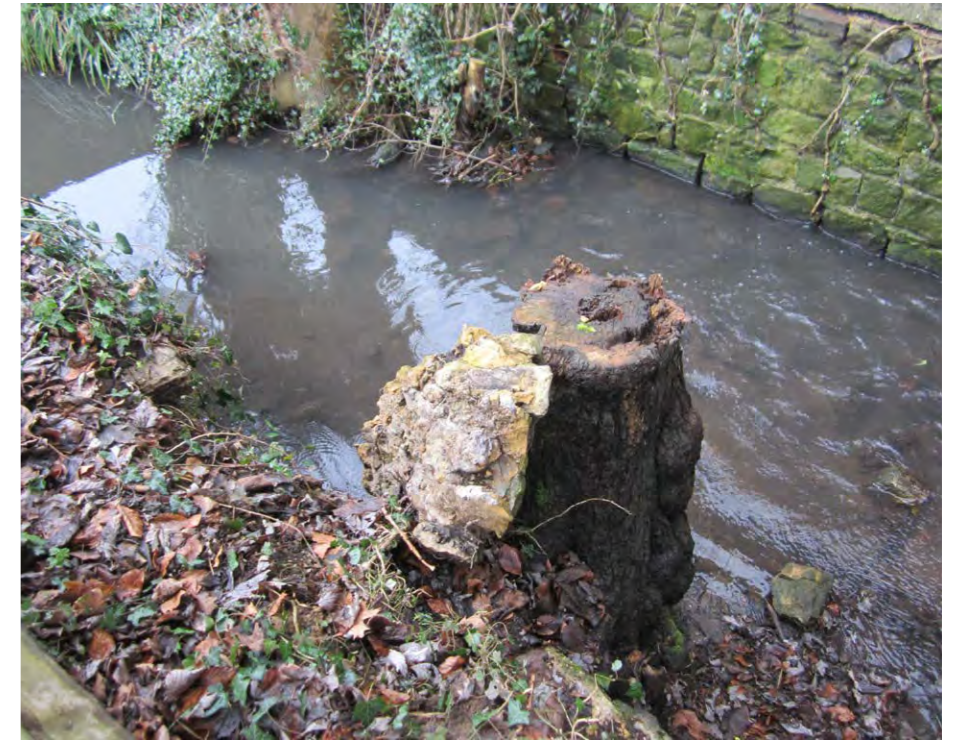
Collapsed stream wall
