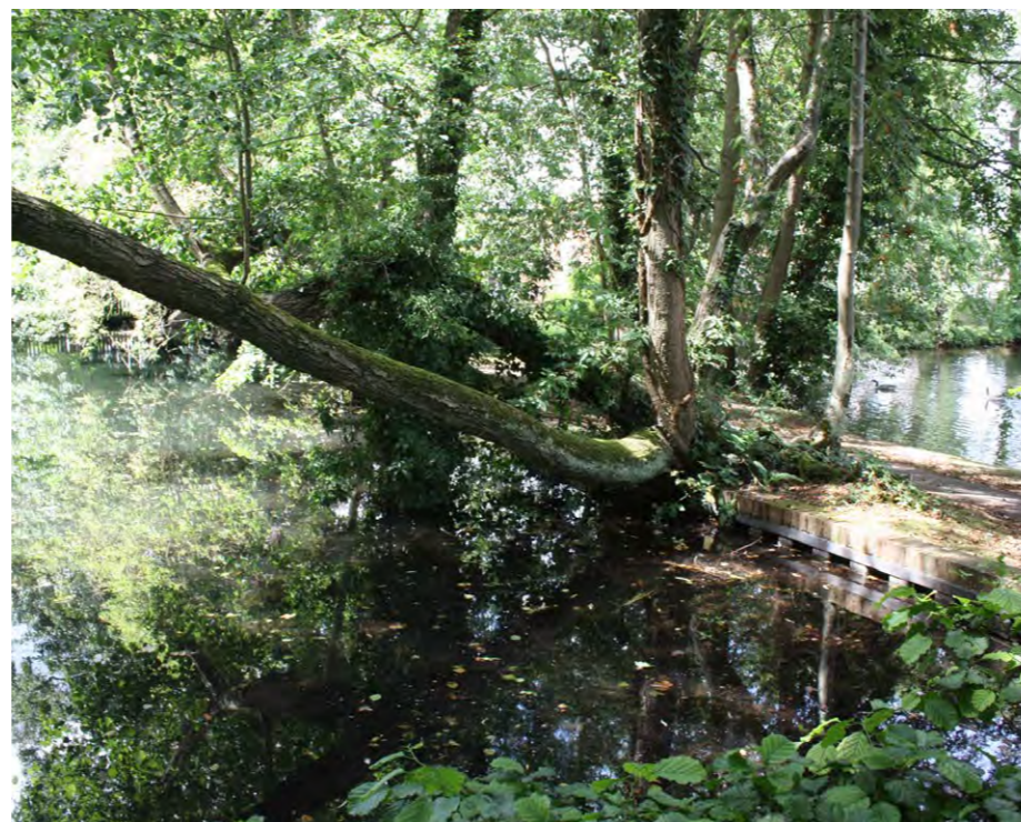
Naturalised trees damaging edges
